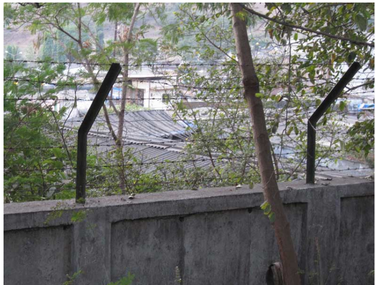
Fig. 3.3 - Part of the Wall on the Thane side of the Park
